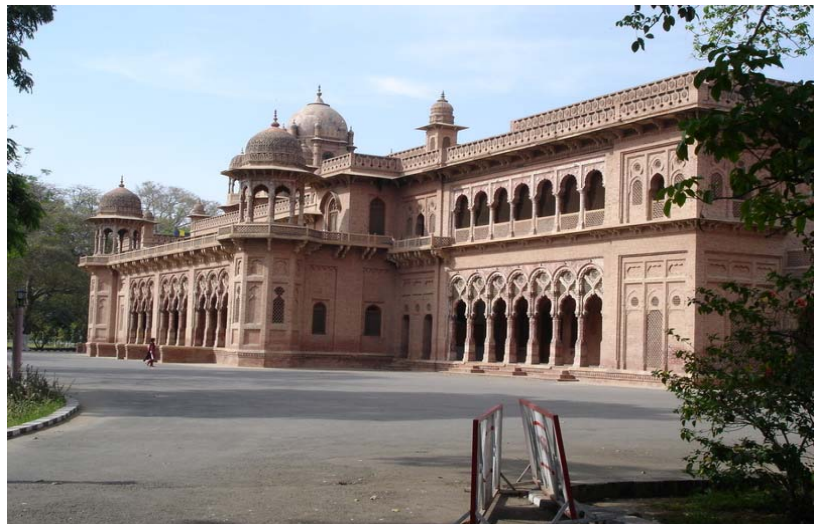
Illustration 6: Aitcheson College, Lahore: Main Building, Southern Façade.
